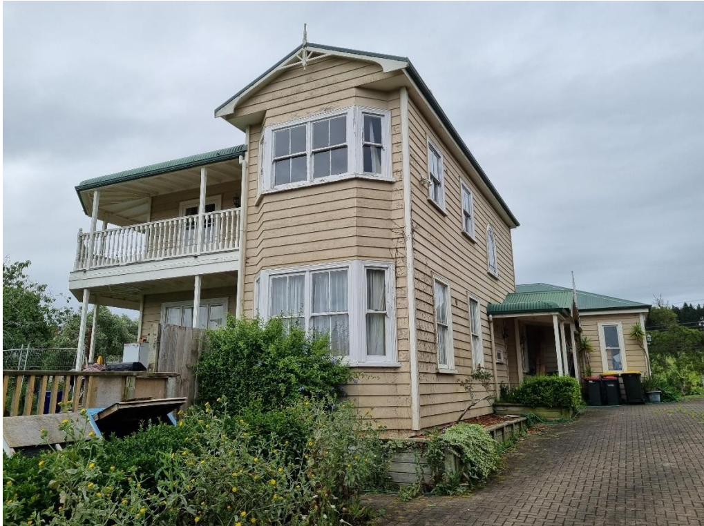
Figure 14. Northern side of building
