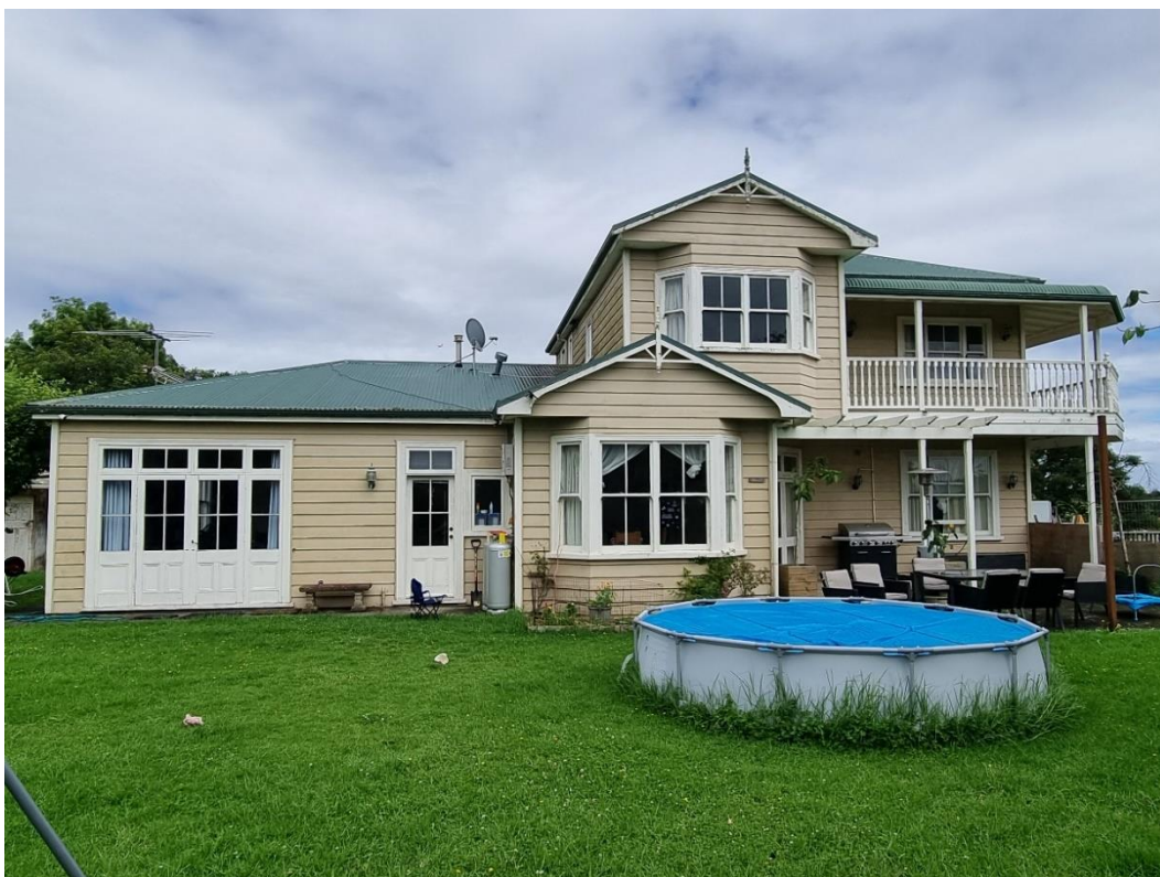
Figure 13. Eastern side of the building
