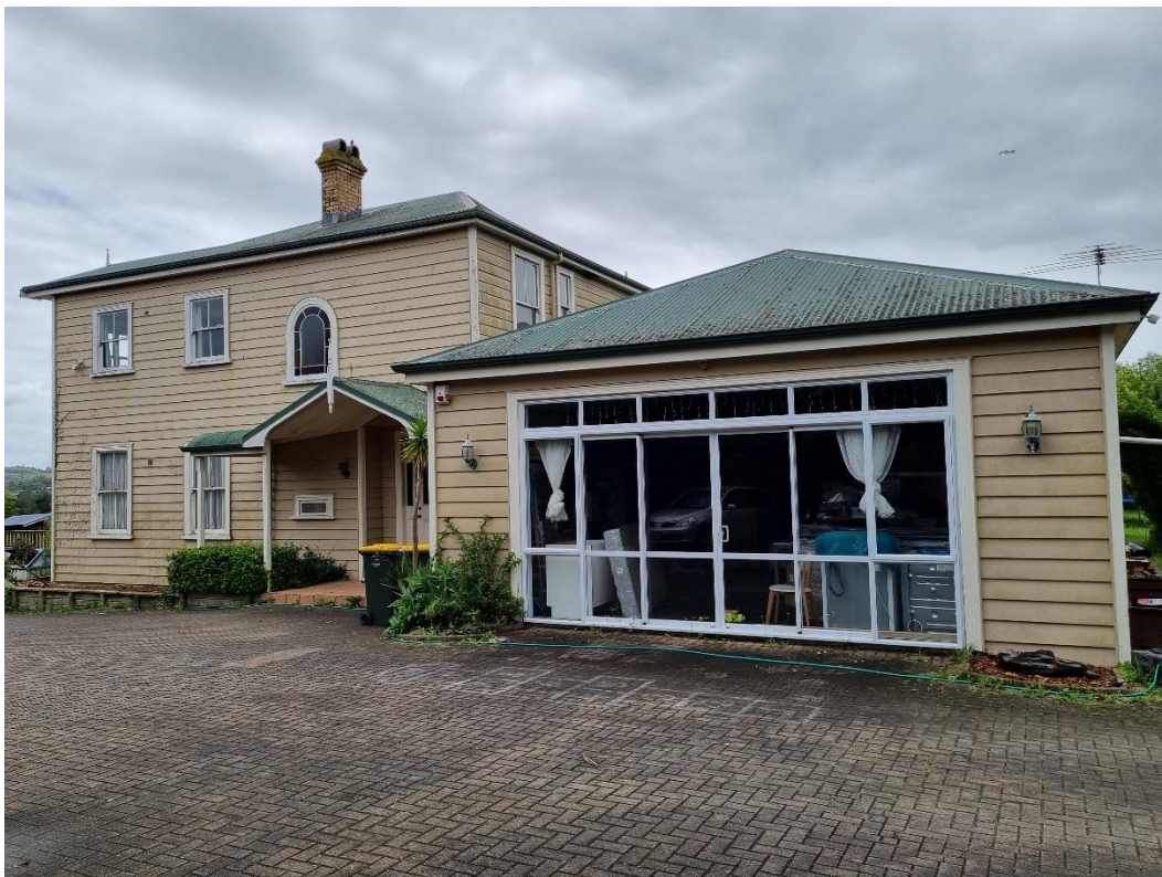
Figure 12. Western side of the house showing modern attachment on right
